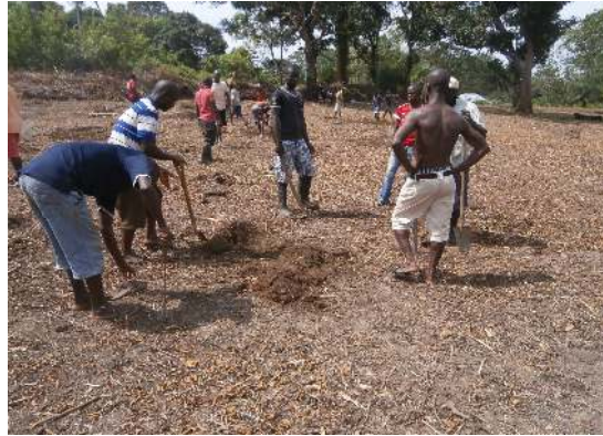
Site clearing and stumping
