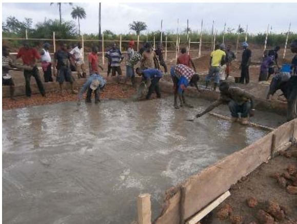
Concreting of tent area
