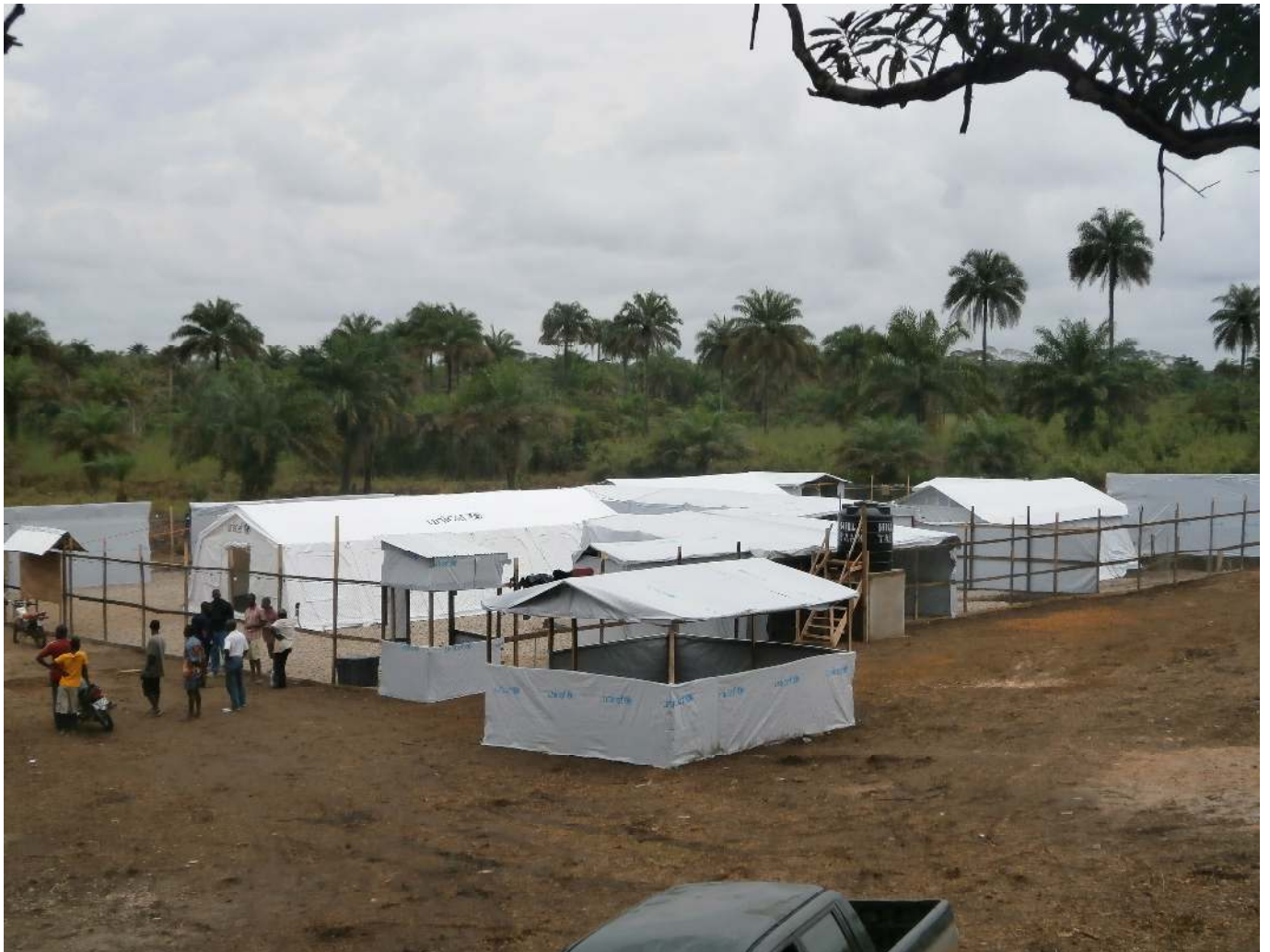
Arial view of the constructed CCC
