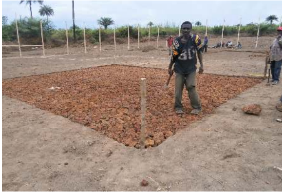
Compacted ground with hard core
