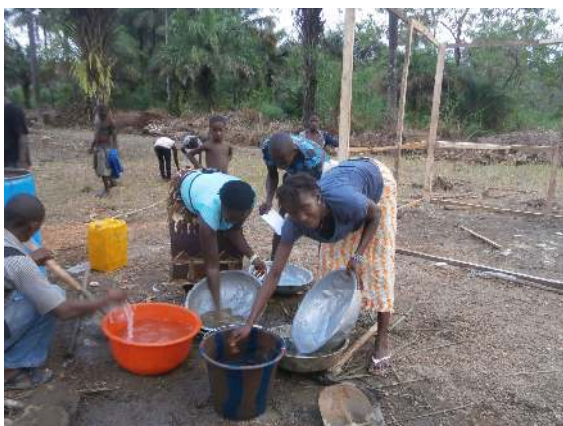
Women participation in CCC construction
